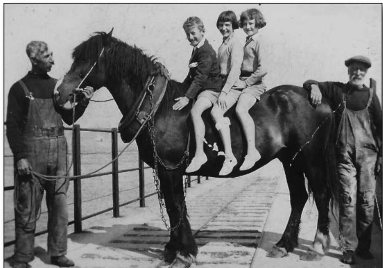
Upper: The pier rails and bogey. The traces of a second railway can be seen on the left, possibly one used during construction.
