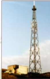
Glengorm transmitter on the hill of Mull
