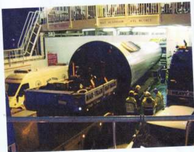
▲ Loading components and handling equipment for the erection of Tiree's wind turbine. Image: Charles McCurdy
