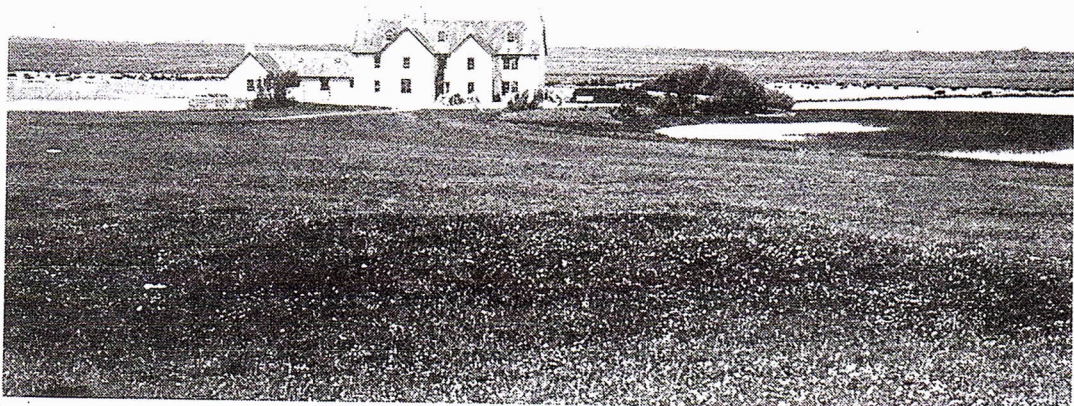
ISLAND HOUSE The Factor's Residence as it looked at the time of the agitation
